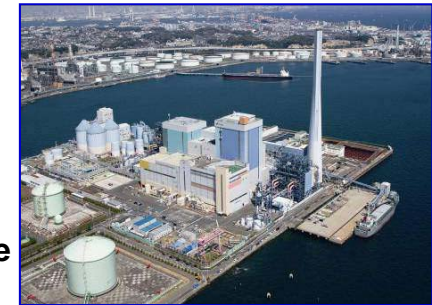
J-POWER Isogo Thermal Power Plant Photo Credit: J-POWER
